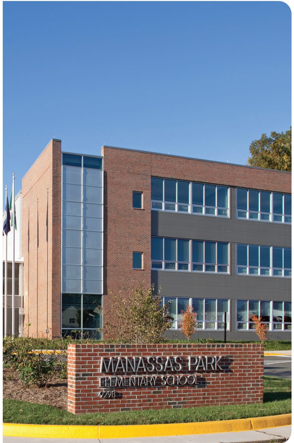
MPES, the first green school in Manassas, was designed with Solarban® 70 glass by Vitro Architectural Glass (formerly PPG glass) to maximize visible light transmittance and solar control
