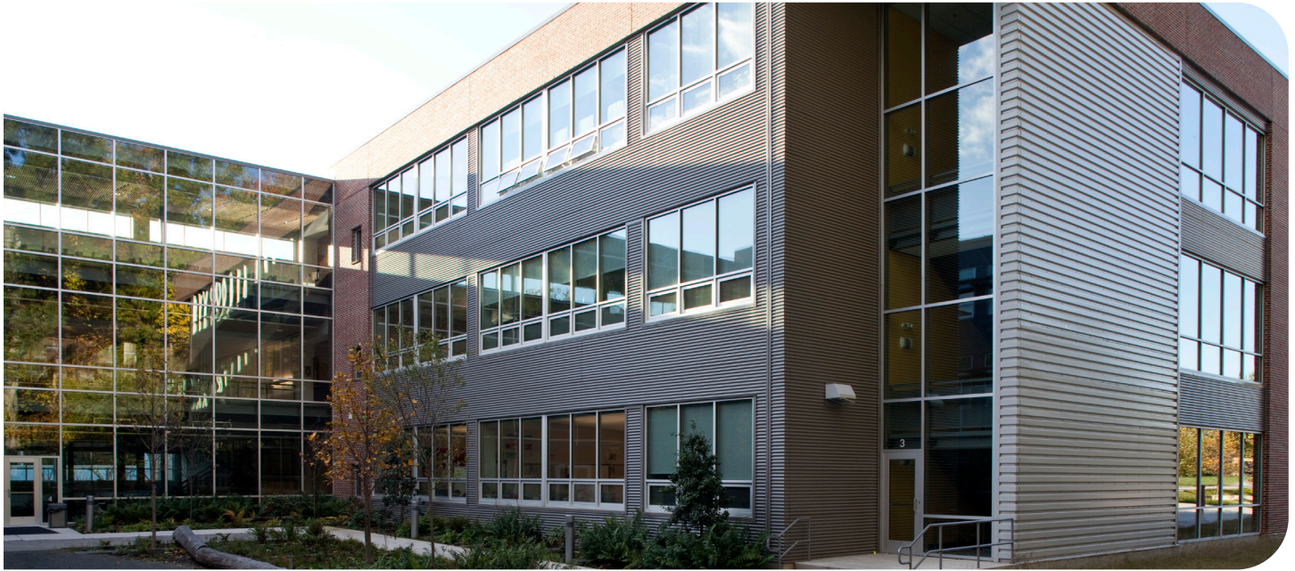
The first LEED®-certified building in Manassas, MPES was also recognized by AIA Committee on the Environment as one of the country's top green building projects of 2009.
